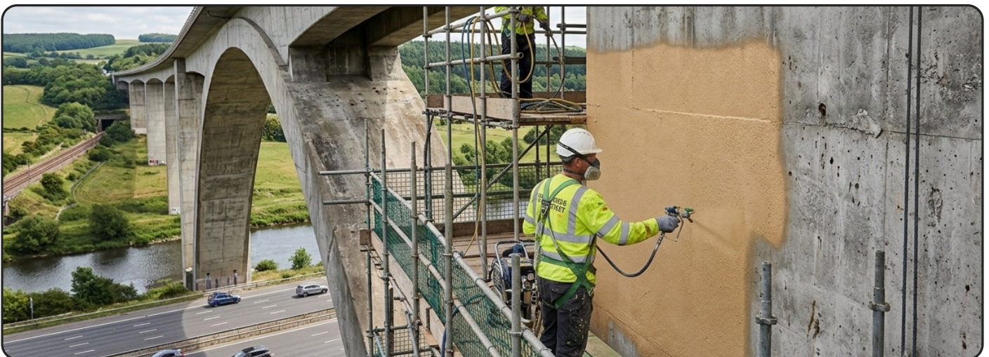
ProTek-Crete applied to a concrete bridge structure - Sandstone finish shown
